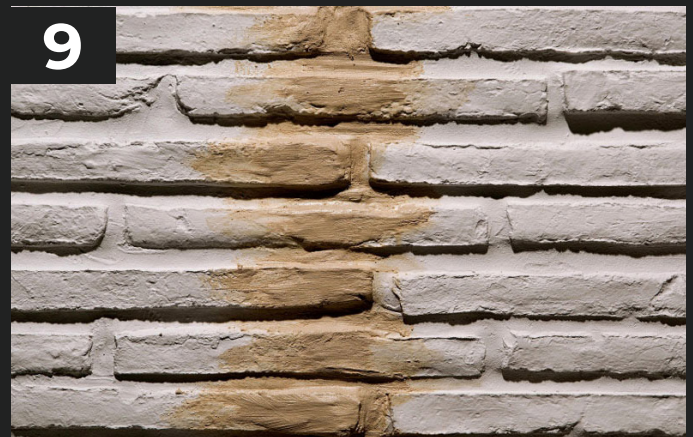
9. Spachtelmasse trocknen lassen Waiting for drying for assembly putty
